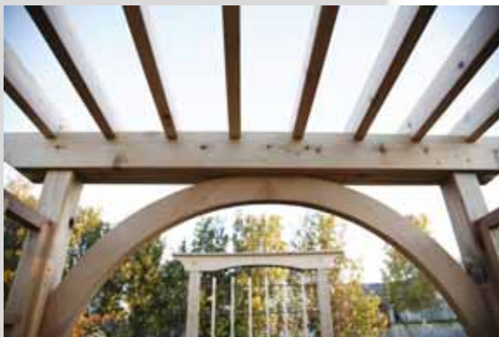
The top members are carefully notched to fit over the cross beams.
