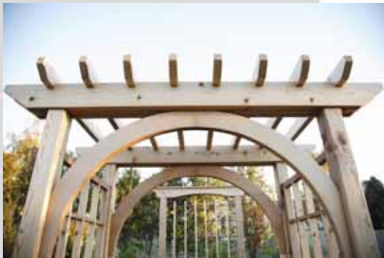
The top members are carefully notched to fit over the cross beams.
