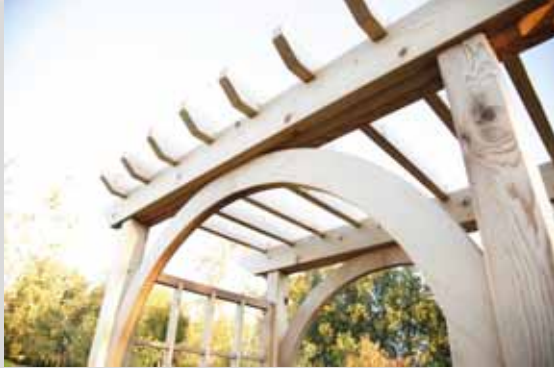
The arches were cut from cedar dimension lumber.
