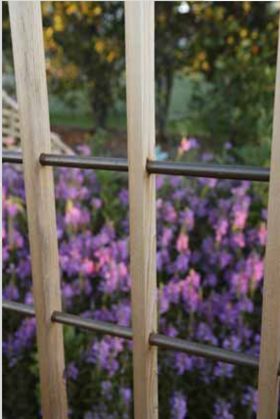
Copper pipe was cut to fit, and the cedar uprights were precisely drilled to receive the pipes. Through only one summer, the pipes have already begun to show their natural patina.
