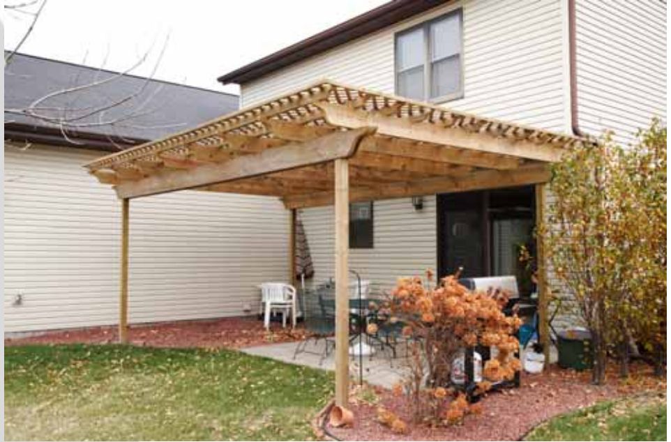
The pergola helps to break up a series of walls that have little glass. The south exposure collects much sunlight and heat. The new pergola shades the patio door and window, allowing filtered light while minimizing glare and excess heat gain into the house.
