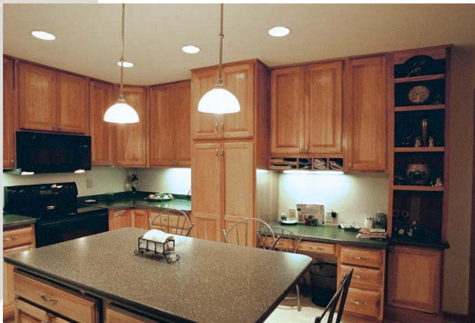
A combination of lighting options allows the space to be fine-tuned for work or for ambience. Fluorescent under-cabinet lights balance the energy usage of halogen recessed cans and incandescent pendants.
