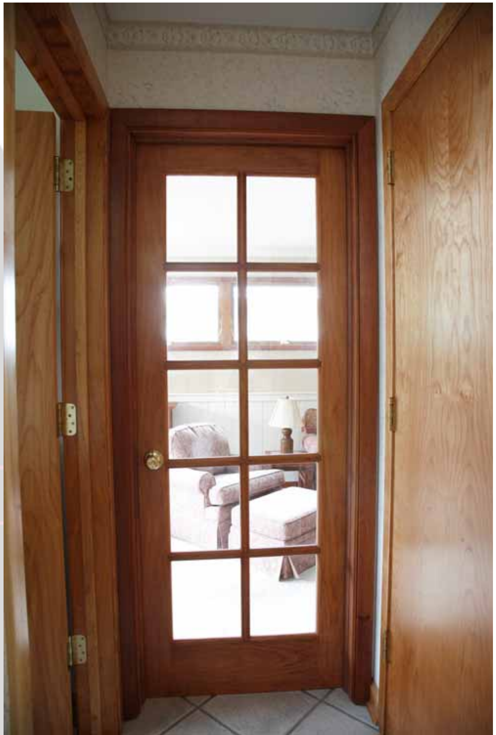
The now-brightened hallway is visible here. The natural light presents the sometimes shiny appearance of the red birch grain at the right moments. The 10-lite door to the family room usually remains open and so was done to match the cherry trim of the family room as seen in the context photos below.
