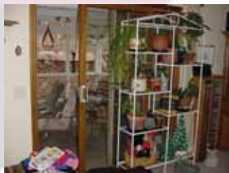
The former screened porch was built on a slab with no footings, and was sinking away from the house. It had low eaves and the interior was simply painted over the structural rafters and sheathing. Low brick side walls were crumbling along with the slab.
