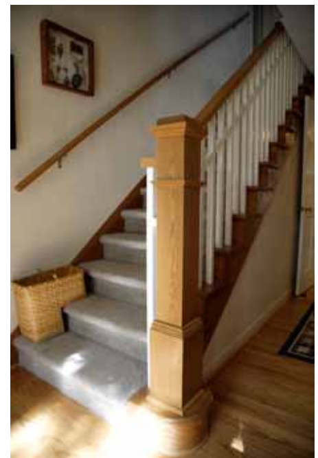
Note the second handrail mounted to the wall. One of the clients utilizes both handrails when traversing the stairs due to knee and back pain. The new system meets building code, functions for the client, and is a beautiful upgrade to the main entry of the home.
