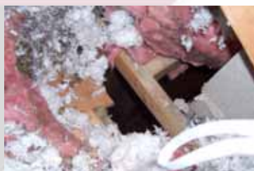
Air leakage through the chimney chase was corrected during the remodel.
